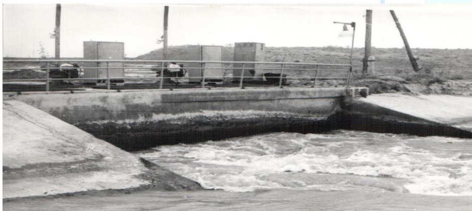
Figure 2. Water intake structure of the Mirishkor Main Canal from the KMC, PC 0+00
